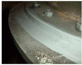
Oily Metal Flange Sealed with Resimac 104 Metal Repair Fluid
