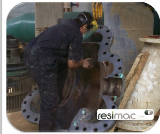
Split Case Pump Volute Repaired and Protected with Resimac 203 SuperFlow
