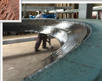
Damaged Turbine Cover Rebuilt with Resimac 204 Heavy Duty and Protected with Resimac 202 Ceramic Repair Fluid
