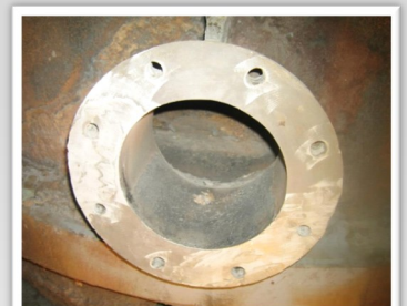
Worn Flange Face Rebuilt and Restored with Resimac 101 Metal Repair Paste
